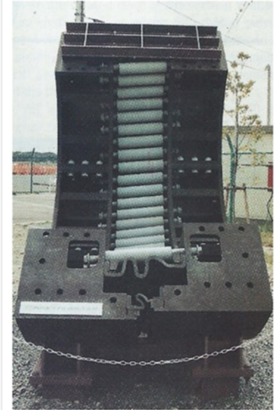
Eight 1.5m wide flexible joint rings are inserted into the primary segmental lining to help the accommodate the settlement and seismic activity
